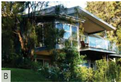
B Residential dwelling at hillside
